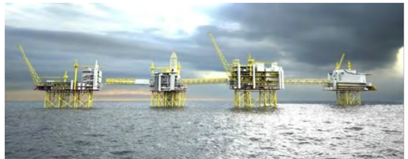
Johan Sverdrup Field Centre in phase 1 with riser platform, drilling platform, process platform and living quarters (Picture: Johan Sverdrup konsekvensutredning)
